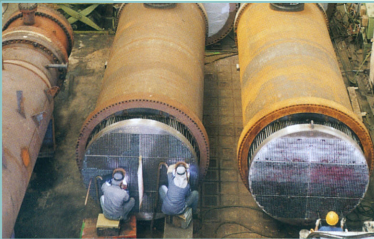
▲機械廠內觀 A View of the Fabrication Shops
