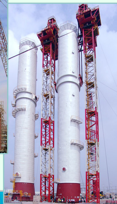
▲C5551/C5552 苛性水洗滌塔 Amin/Caustic Water Wash Tower SA516-70 \phi 7.8 m x 74.6 m L x 1,060 / 1,240 Ton
