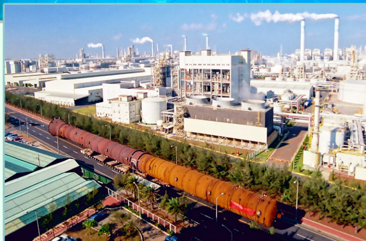
▲C470 乙烯分餾塔 Ethylene Fractionator SA537-CI.1 \phi 5.8 m x 114 m L x 911 Ton
