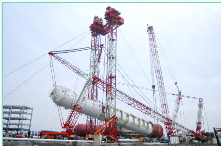
▲C540 丙烯分餾塔 (1 號) Propylene Fractionator NO.1 SA516-70 \phi 7.0 / 8.2 m x 80.5 m L x 1,260 Ton
